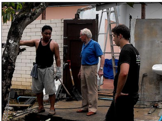
Rommel, John and Alan at the work site the day before the accident.
