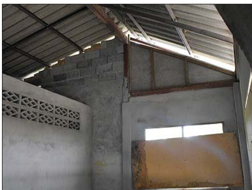
An inside view of portion of the building.
